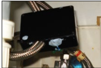
Fig. 2. Sensor mounted at an inflow pipe of a washbasin
